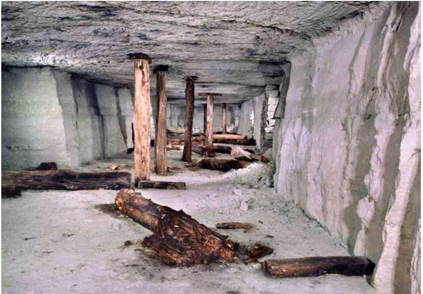
Mined hearthstone gallery at Marden. Almost all the rock was taken out for sale. Spoil is represented by minimal amounts of rock containing chert nodules. Note the irregular gallery walls with wedge marks
